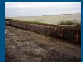
With RDFW, a crew of six laborers and one loader operator can build a wall 100 feet long, four feet wide and four feet high in one hour. An equivalent sandbag wall requires 35 laborers over 19 hours to construct. RDFW is highly cost-competitive with sandbags.
