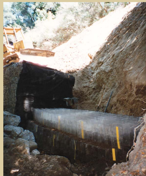
RDFW stream-diversion wall (curved, white object in background) allowed access to construction area. In this case, the wall was 16–24 inches in height, but RDFW stacks as high as six feet.
