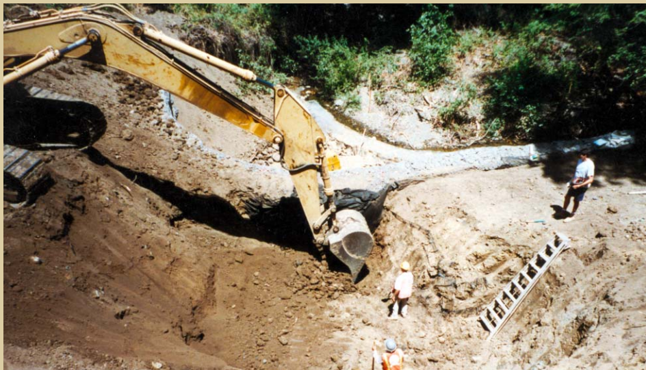
RDFW stream-diversion wall (curved, white object in background) allowed access to construction area. In this case, the wall was 16–24 inches in height, but RDFW stacks as high as six feet.
