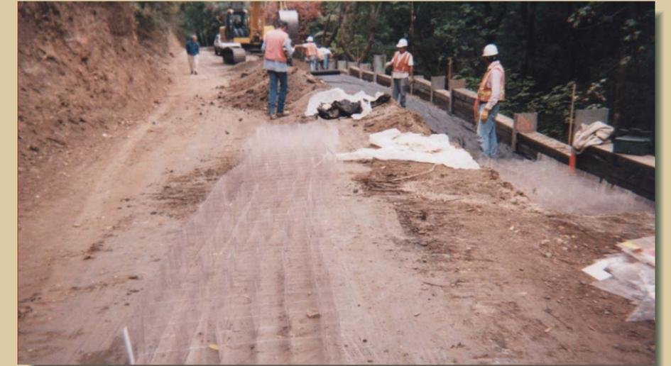
RDFW was used in road shoulder construction. Confined-cell geosynthetics (geocells) can provide the same load-bearing strength as much thicker rock-filled base.
