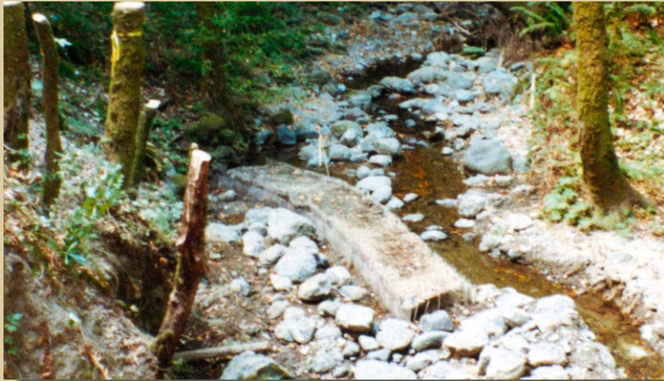
A stream-diversion wall was constructed using Geocell Systems' RDFW. Unlike other geocellular materials, RDFW can be stacked to form walls for water diversion or retention.
