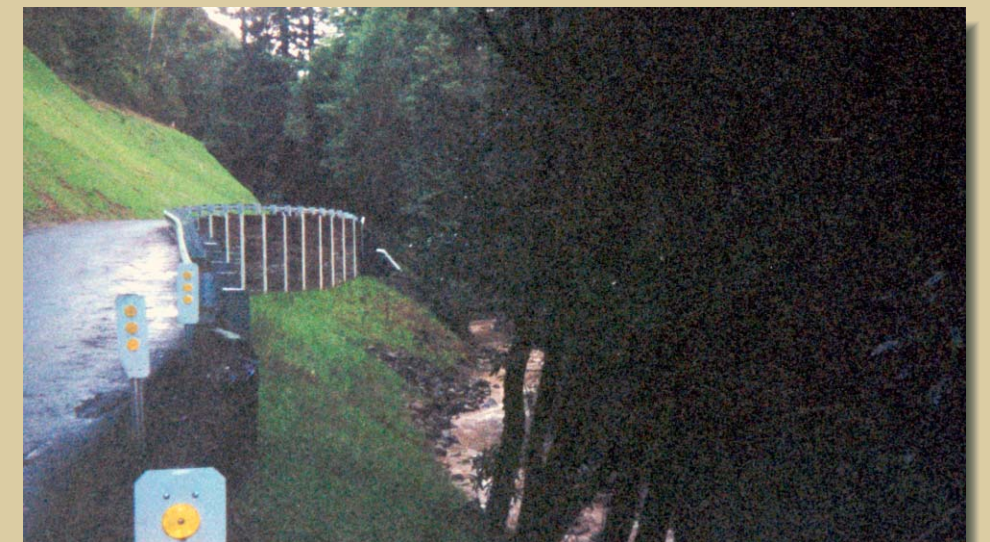
RDFW was used extensively in the repair of Alpine Road.
