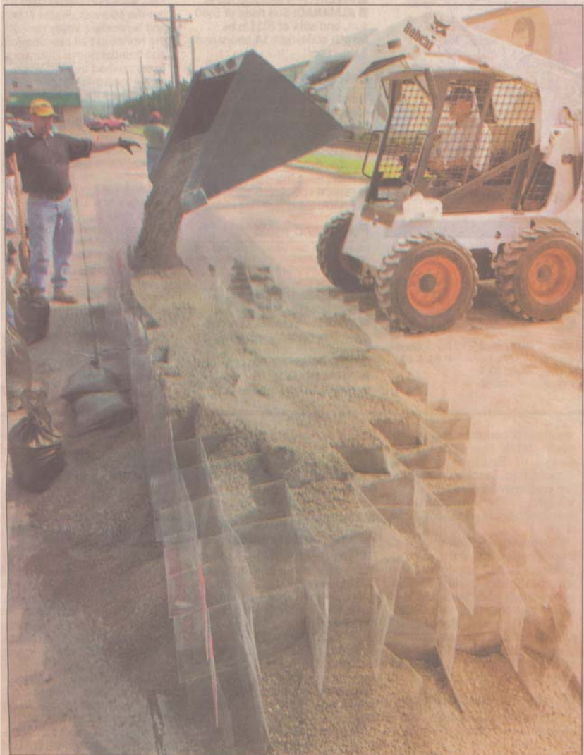
Representatives of Geocell Systems and Spartech Plastics demonstrated the Rapid Deployment Floodwall in the Main Street parking lot in downtown Cape Girardeau Tuesday.
