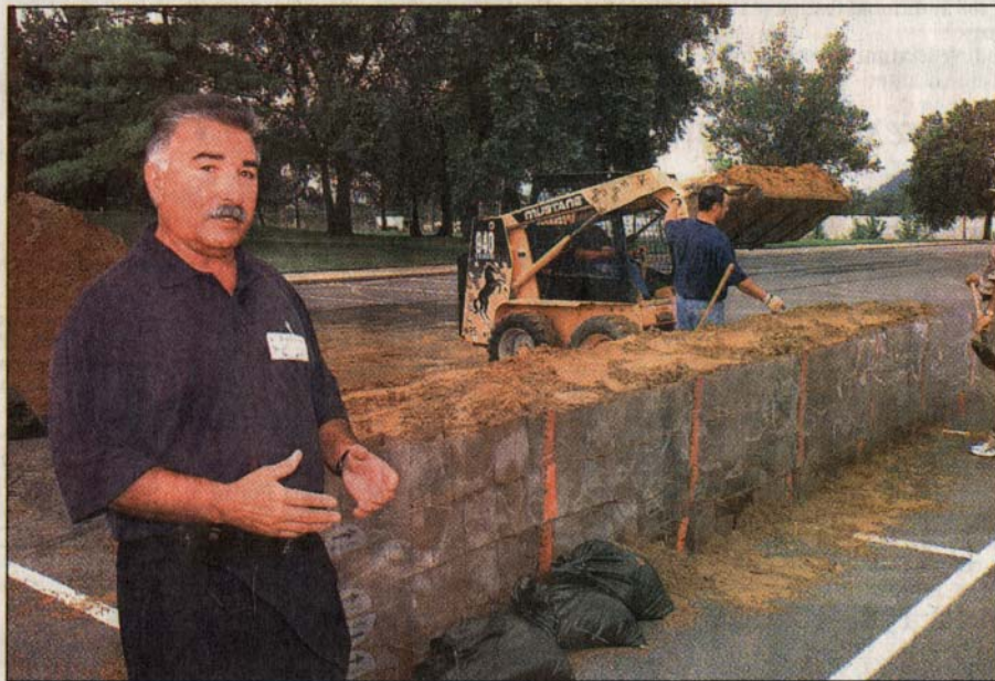
Al Arellanes, president of Geocell Systems, explains the new Rapid Deployment Flood Wall that his company and Spartech Corp. have developed in partnership with Eastman Chemical Co.
