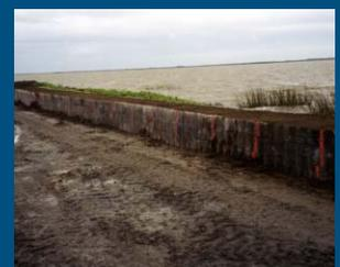
*With RDFW, a crew of six laborers and one loader operator can build a wall 100 feet long, four feet wide and four feet high in one hour. An equivalent sandbag wall requires 35 laborers over 19 hours to construct.*
