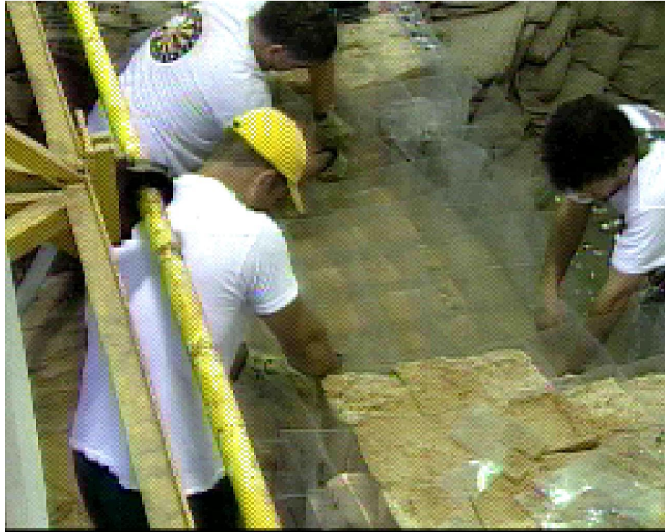
Figure 30. Repair of damaged Section 1 in the wet, d = 24 in.
