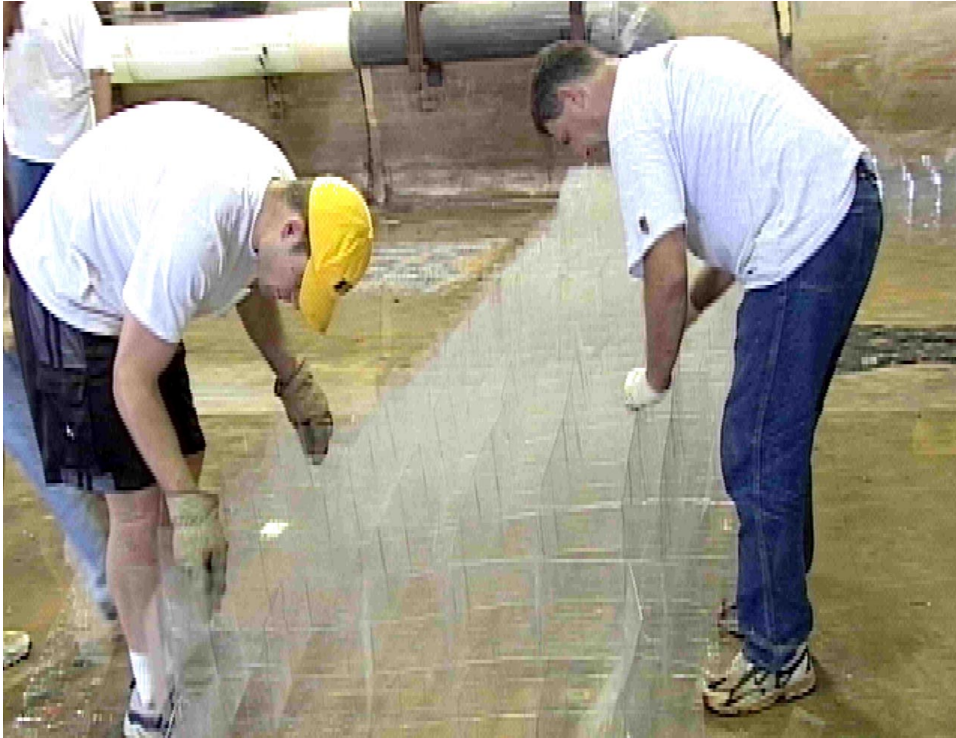
Figure 7. Stacking and interlocking of RDFW grids
